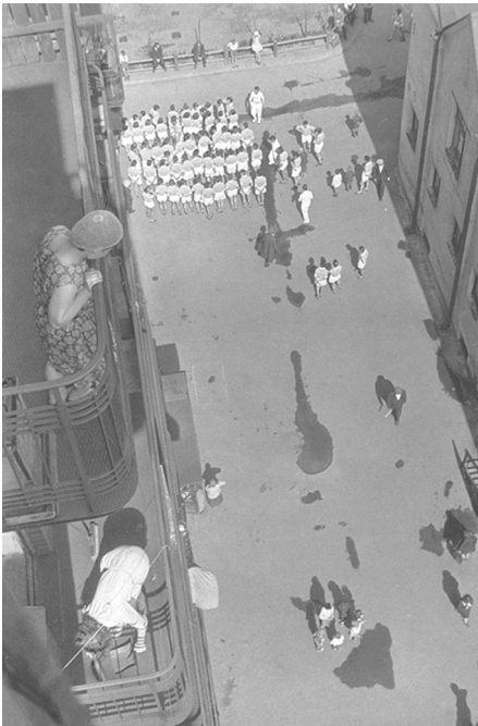
Figure 36 Alexander Rodchenko, Shorka dlya dyemonstratsii (Assembling for a Demonstration, 1928). Photograph taken with a Leica from a balcony. Like Moholy-Nagy, Rodchenko thought that viewing the modern city required unusual angles. Much of his work as a photographer went into demonstrating that compositional skill and experimental shot-angles not only made photography a modern artform in its own right but also allowed people to see the world differently.
